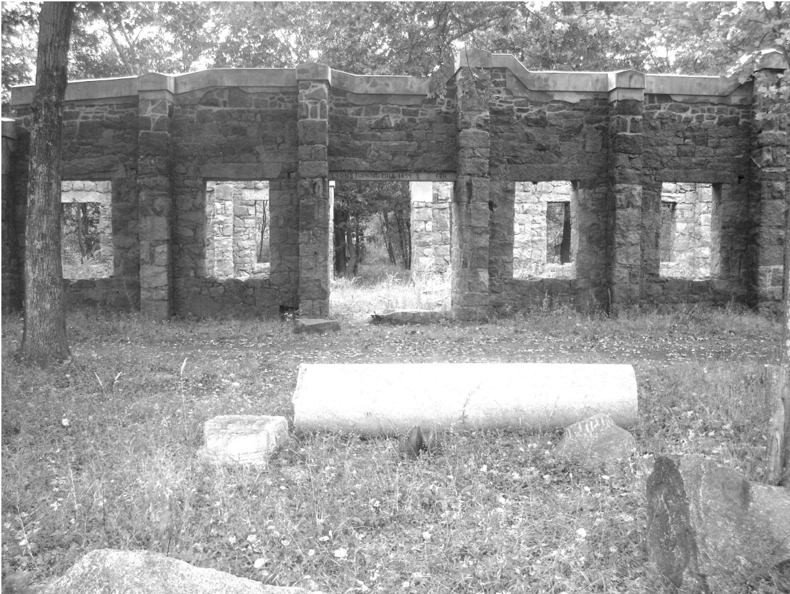
Lyons Turning Mill center doors that would let a rail car pass through to be loaded or unloaded by the 20 ton overhead traveling crane. Photo by Tom Bonomi 2013
